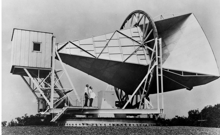
**Figure 26:** The Holmdel Horn Antenna in use in 1962 by Penzias and Wilson.
