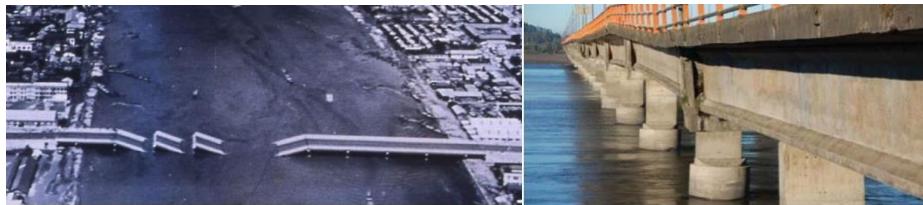
Figure 1: Left-Showa Bridge after 1964 Niigata earthquake (Bhattacharya et al., 2014); Right-Juan Pablo II Bridge after 2010 Chile earthquake (Kawashima et al., 2011)
