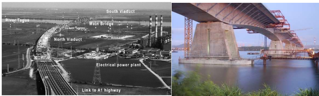
Figure 10 - Leziria Bridge under construction
