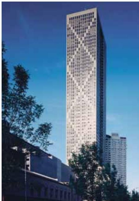
*Onterie Center. The strength of the building's structural system is expressed in its facade. Courtesy of SOM.*
