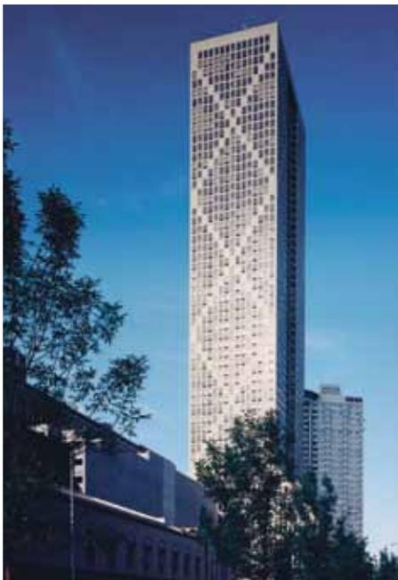
*Onterie Center. The strength of the building's structural system is expressed in its facade. Courtesy of SOM.*
