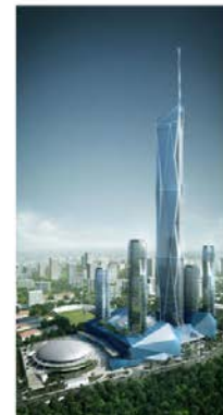
A rendering of megatall skyscraper Merdeka PNB 118, currently under construction in Kuala Lumpur, Malaysia. (Image courtesy of SawTeen See/LERA Consulting Structural Engineers)
