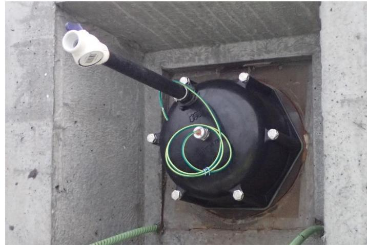
Measuring cable through cap
