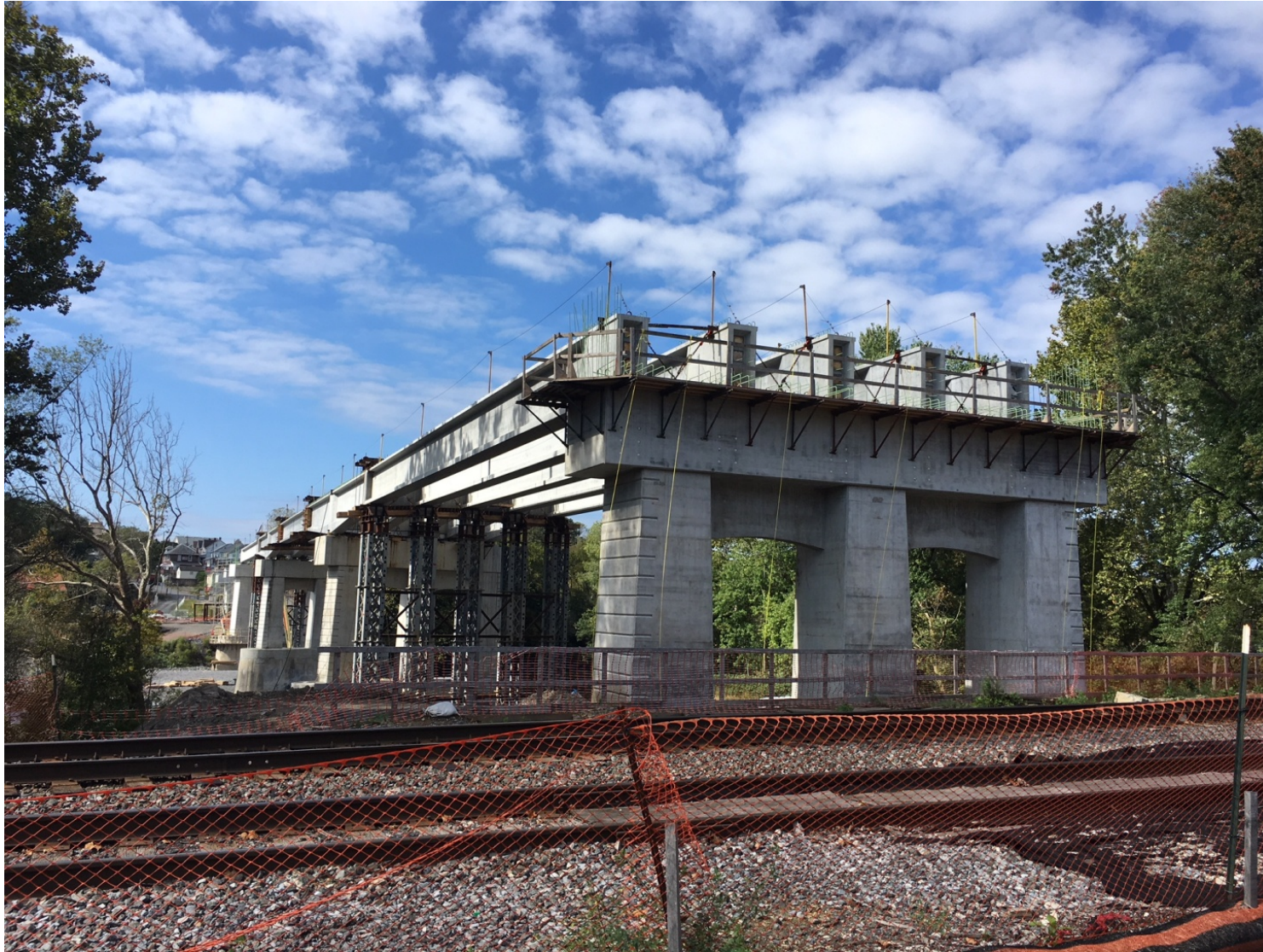
Lehigh University EIT Workshop: Coplay Bridge Demonstration Project – October 24 th 2018
