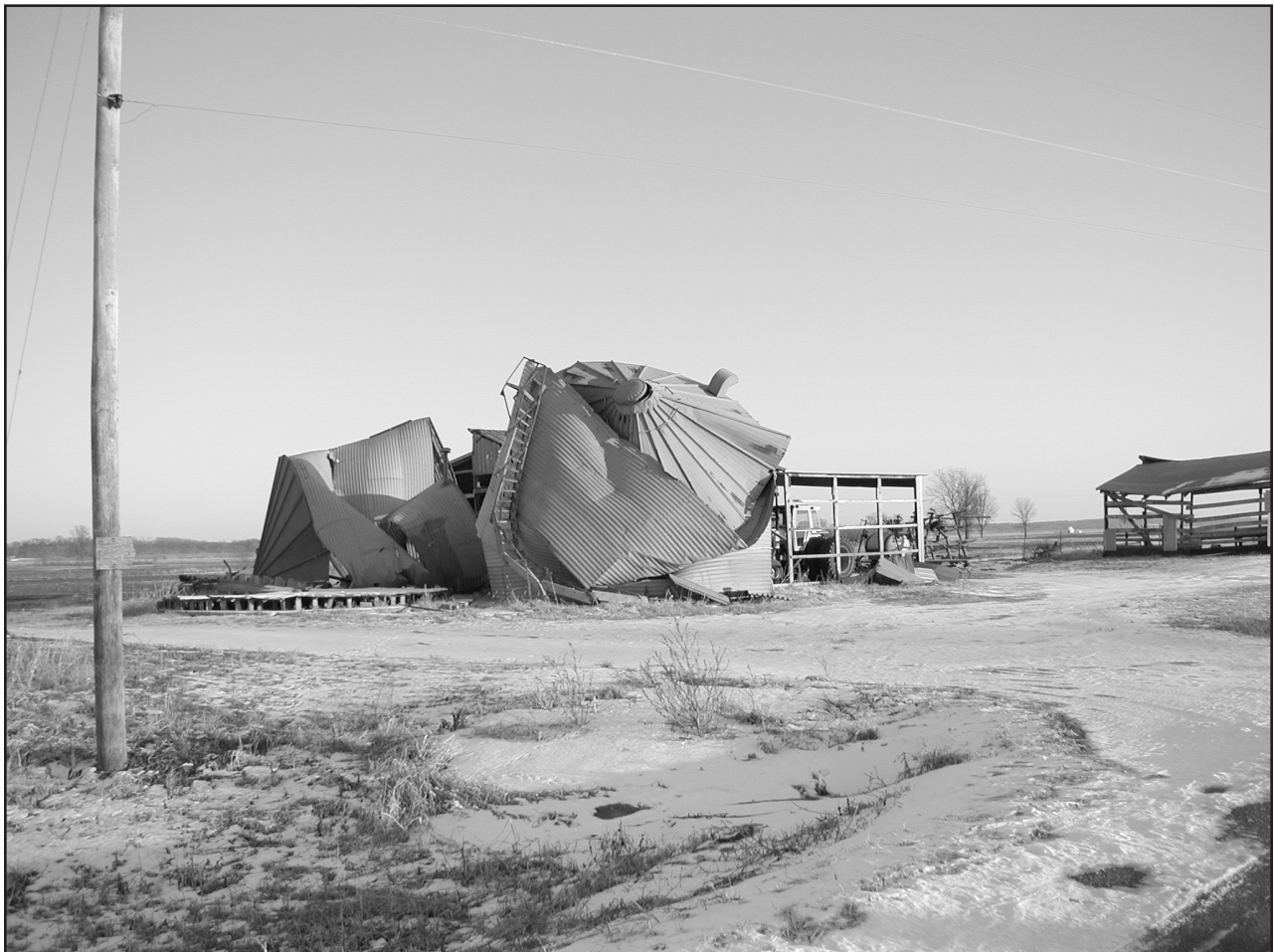
Figure 3. Flood-damaged grain bins in the Warsaw Bottoms six months after the flood (photo: D. Casagrande).
