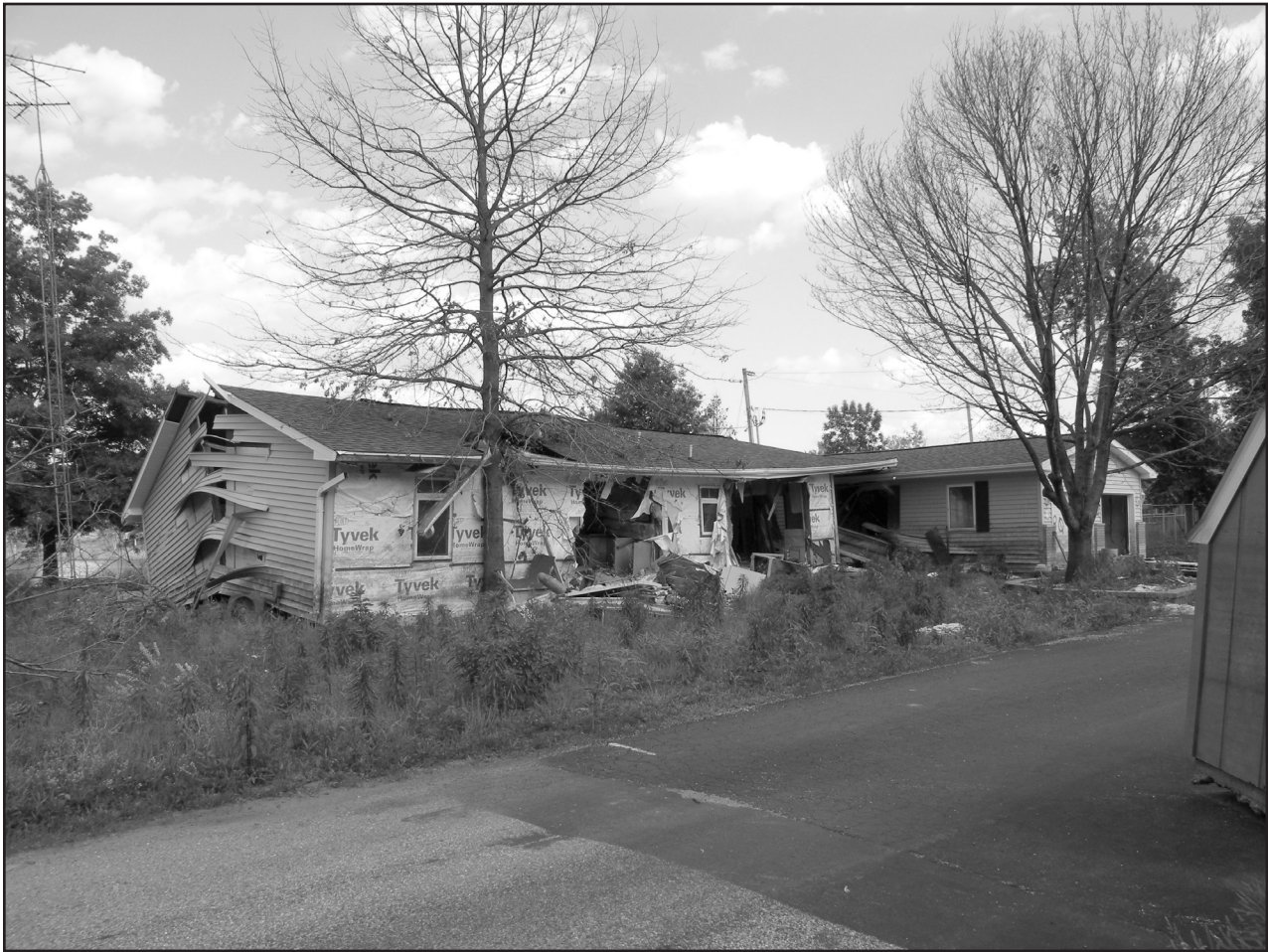
Figure 2. Flood damaged house near Gulfport, Illinois (photo: D. Casagrande).
