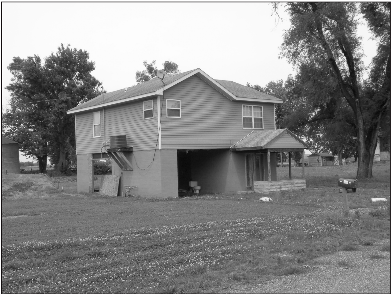
Figure 4. Repaired elevated house in Meyer, Illinois two years after the flood (photo: D. Casagrande).
