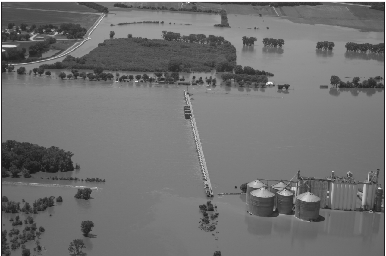
Figure 1. Aerial view of the Canton dam (Lock and Dam No. 20) with breached levees in Meyer, Illinois (photo: Nathon Fox).
