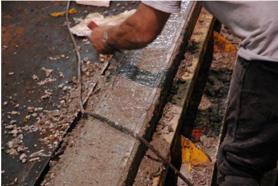
Figure 7-12: Applying the Rake Surface Finish
