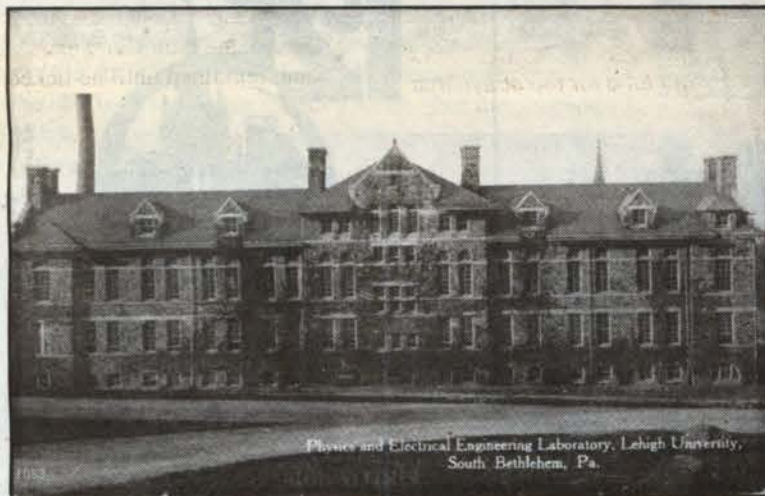
A postcard from about 1910 shows the rebuilt structure. The central tower was eliminated. The new building had three, rather than four stories, according to the Brown and White.
