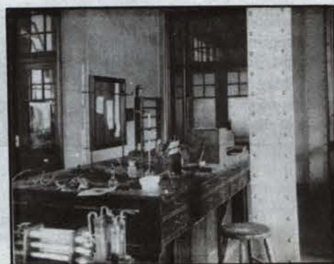
One of the chemistry labs about 1890. The iron beams, which can still be seen inside the building, were used to support the weight of the structure.
