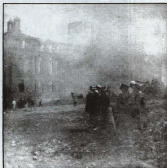
Only the outer walls remained after the roof fell into the ruined building.
