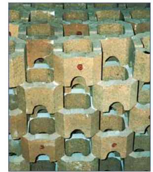
Typical regenerator chimney block packing during construction
