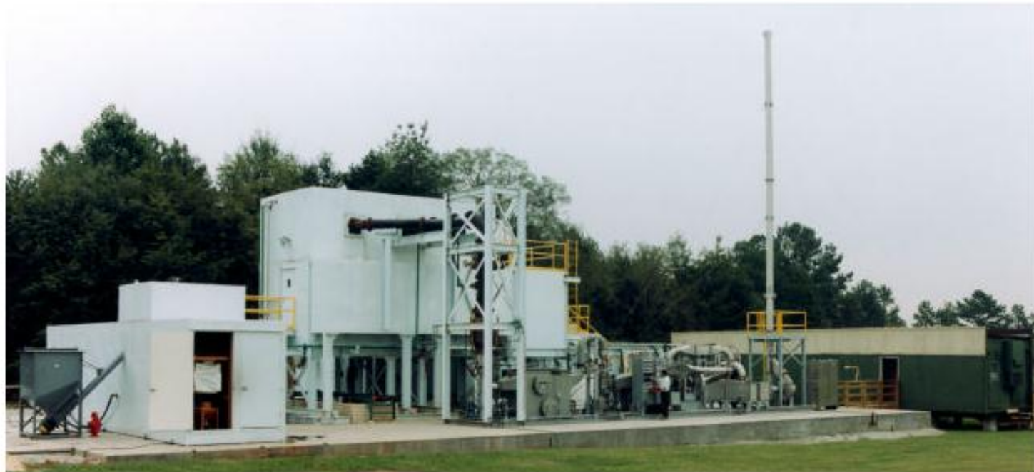
Transportable Vitrification System (TVS) in the field. Composed of 5 modules , a feed batch preparation module (left) with an exterior waste tank or hopper, a melter module (center double story), an off-gas module (along front face of concrete pad with a 40 foot tall off-gas stack), a control/power supply module (behind the off-gas and melter module). Co-designed by EnVitco Corporation and SRTC [24].
