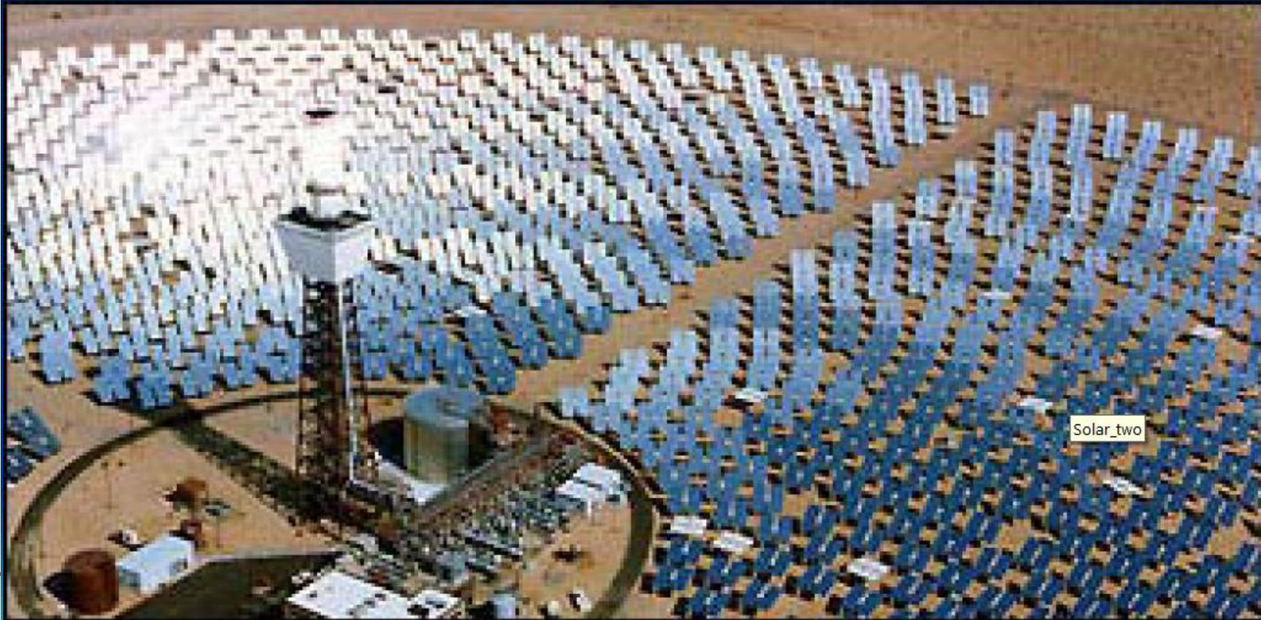
In **tower (heliostat)** receivers, the temperature can reach more than 1000 °C, allowing in principle **higher efficiency rates of energy conversion**. The high temperature (metal or ceramic) **receivers** are **covered by** a cooled **silica glass window** in this case, where porous silica **quarter wave AR coatings** are also used.
