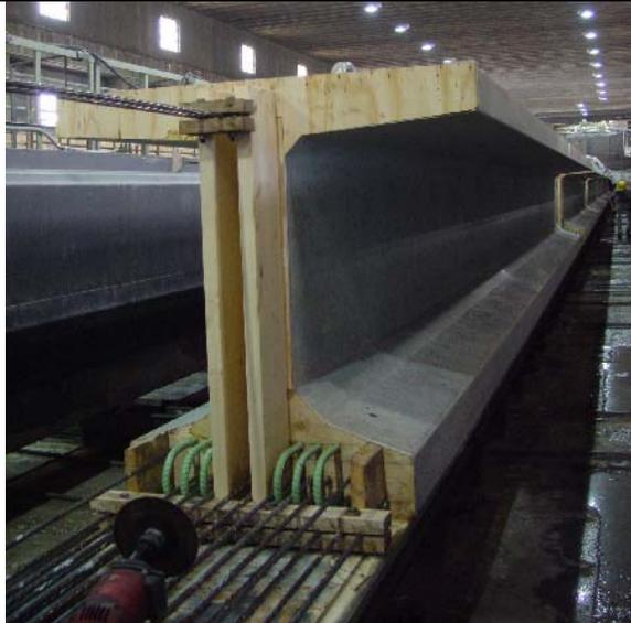
11) Cover and heat beams with radiant heat for initial cure period (~24 hours). Open forms on completion of cure
