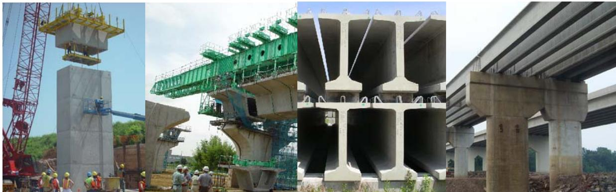
a) Precast piers      b) Precast box segments      c) Prestressed bulb beams      d) Prestressed superstructure
