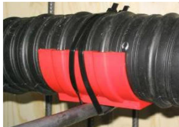
Figure 21. Protecting half shells to support the duct at high curvatures; a) metal half-shell and steel tying wires, b), plastic half-shell and plastic tying wires. Note that for PL2 and PL3, metal half-shells and steel tying wires are not allowed [3, 4].
