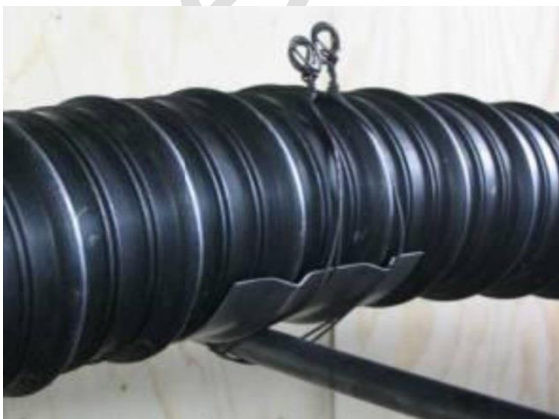
Figure 21. Protecting half shells to support the duct at high curvatures; a) metal half-shell and steel tying wires, b), plastic half-shell and plastic tying wires. Note that for PL2 and PL3, metal half-shells and steel tying wires are not allowed [3, 4].
