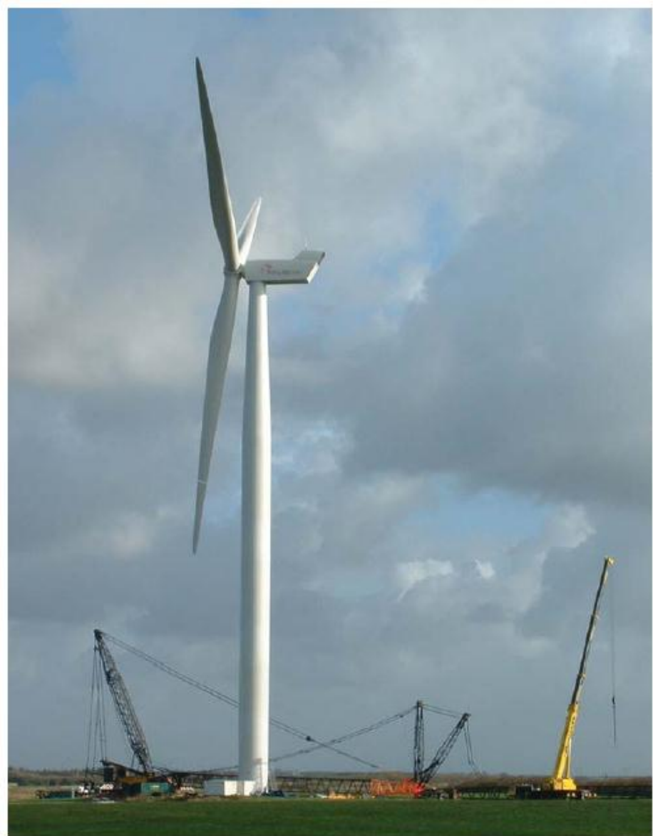
Figure 1 The world's largest wind turbine (summer 2004) at Risoe National Laboratory test site, Høvsøre, Denmark. Tower height is 120 m , rotor diameter is 110 m , and generator power is 3.6 MW.
