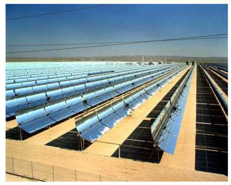
Parabolic trough technology for CSP
