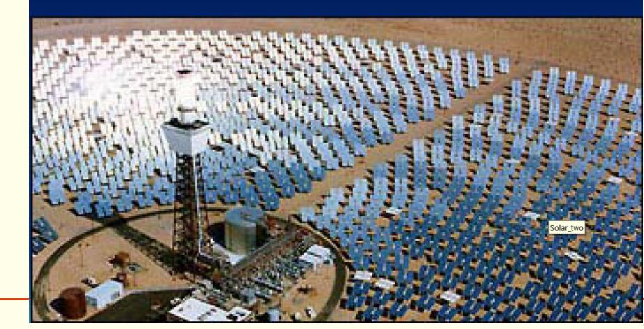
In tower (heliostat) receivers, the temperature can reach more than 1000 °C, allowing in principle higher efficiency rates of energy conversion. The high temperature (metal or ceramic) receivers are covered by a cooled silica glass window in this case, where porous silica **quarter wave AR coatings** are also used.
